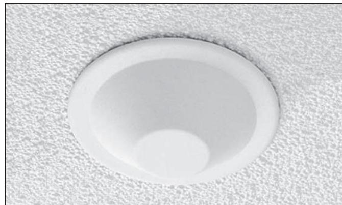
When the ceiling temperature rises, the solder holding the cover plate melts, allowing the release of this part and thus exposing the Model F1FR-300 QREC sprinkler inside to the rising ambient temperature.
