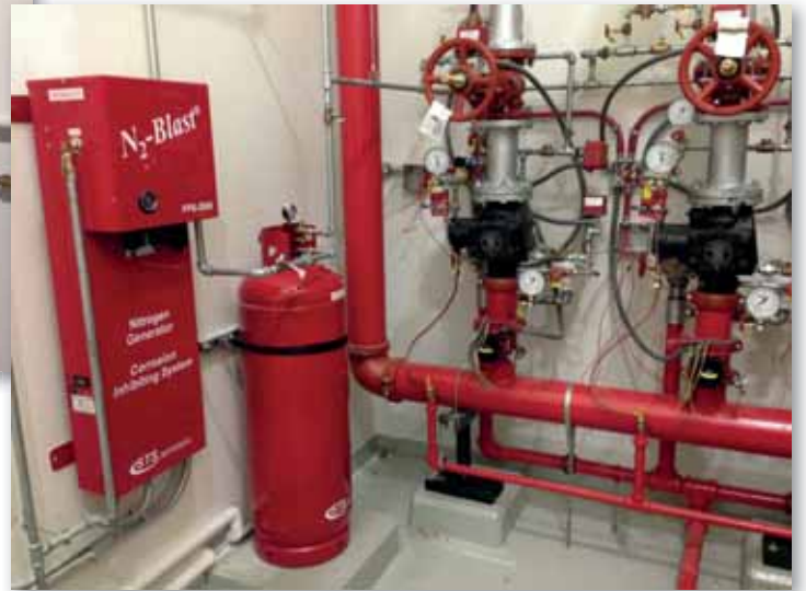
South-Tek N 2 -Blast® Nitrogen Generator fitted to a Reliable Model DDX PrePak Preaction System and Model DDX Preaction Valve.
