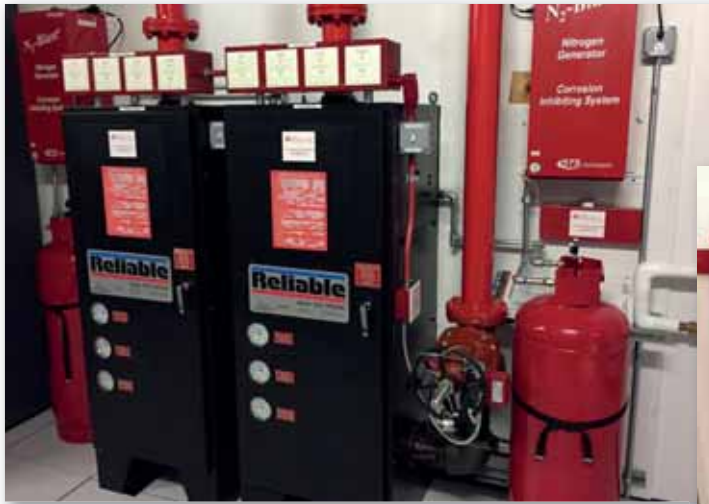
South-Tek N 2 -Blast® Nitrogen Generator fitted to a Reliable Model DDX PrePak Preaction System and Model DDX Preaction Valve.
