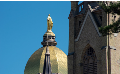
Dry Pipe Valve in Basilica Basement (top), PrePaK (middle), Deluge Systems protect the Golden Dome and bell tower (bottom)
