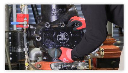
3. Remove the bolts from the striker plate assembly using the provided Allen wrench.
