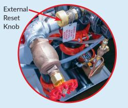
Resetting the clapper of the Model DDX Deluge Valve is easily accomplished using the external reset knob at the rear of the valve.
