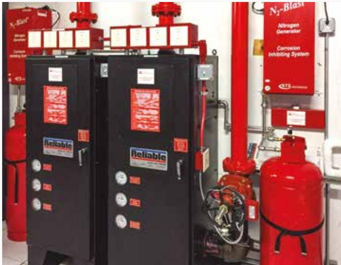
South-Tek N<sub>2</sub>-Blast® Nitrogen Generator fitted to a Reliable Model DDX PrePak Preaction System and Model DDX Preaction Valve.
