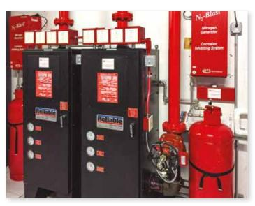
South-Tek N<sub>2</sub>-Blast® Nitrogen Generator fitted to a Reliable Model DDX PrePak Preaction System and Model DDX Preaction Valve.
