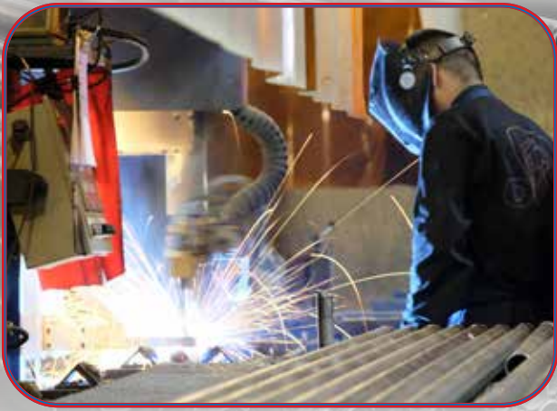
Pipe Fabrication facilities open (2006)
