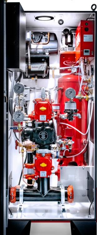
Reliable® PrePaK™ systems are cabinet-enclosed, factory-assembled preaction, dry, and deluge systems.
