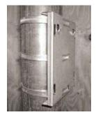
Ensure that the hooks are at the top when installed and that all three straps are fastened tight against the riser (no slack).
