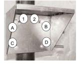
**1 & 2** - Use the rectangular holes on the bracket to rest it on the riser plate hooks.
