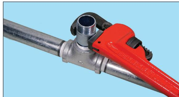
3. Apply PTFE tape or thread sealant to the thread of Inlet Nipple in accordance with the PTFE tape or thread sealant manufacturer's instruction and NFPA 13 guidelines. Use a pipe wrench to install the Inlet Nipple to the branch line as seen on above picture. The Torque Range should be approximately 44 ft/lbs, approximately 1/2 to 3/4 turn past hand tight. **Apply torque only to the Nut and Do NOT surpass the recommended torque.**
