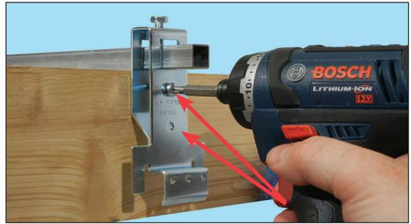
5. Once in place, secure the bracket assembly to the wood beam ceiling grid by using four (4), #8 x 2” ~ 3” wood screws through the holes provided on each side of bracket. On each side of the side brackets, there are two (2) holes for self-drilling sheet metal screws as shown above. Make sure to use both holes to secure the side brackets firmly. Ensure that the wood screws penetrate the wood beam ceiling grid until side bracket is securely in place.
