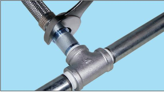
4. Install Outlet Nipple to the Nut of the Flexible Hose by using a pipe wrench. The torque range should be approximately 44 ft/lbs, approximately 1/2 to 3/4 turn past hand tight.
