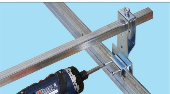
7. Once the Bracket Assembly is properly positioned, hold bracket in place and secure bracket to T-Bar grid using a screw driver and enclosed screw and bolt. Tighten the bolt first with a torque of 2.24 ft/lbs and tighten the screw bracket is fully secured.
