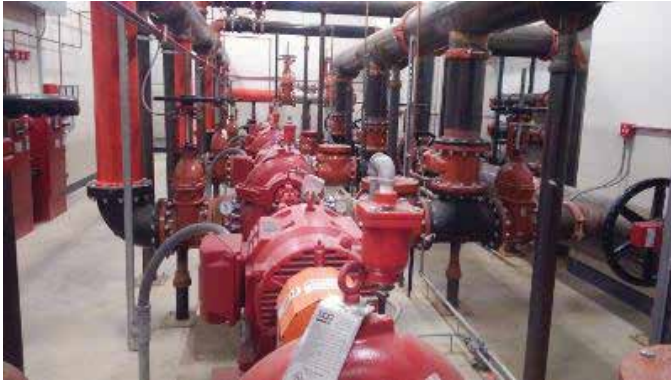
Four 2,500 gpm electric fire pumps were installed and supplied by a new 16" ductile feed into the building.
