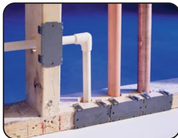
No tools are required for this press-on protection plate. See page 105
